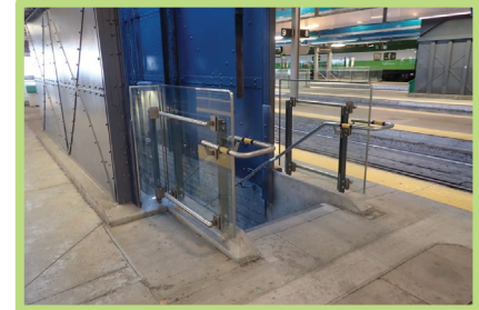
Representative photo of heritage elevator enclosure converted to a stair.
