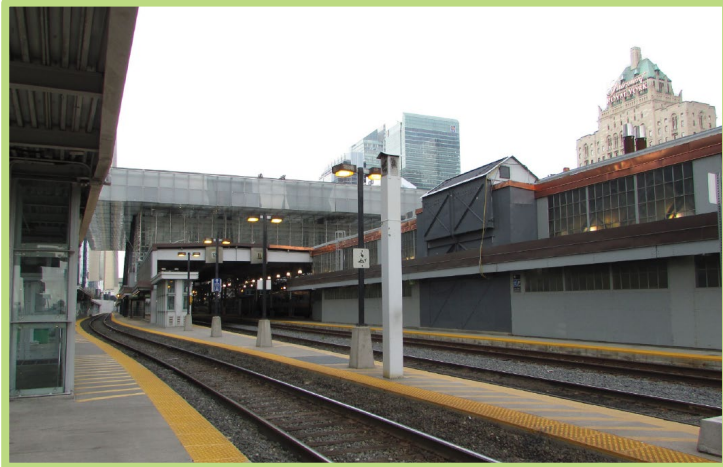
Existing view of Platform 20/21 from Platform 26/27
