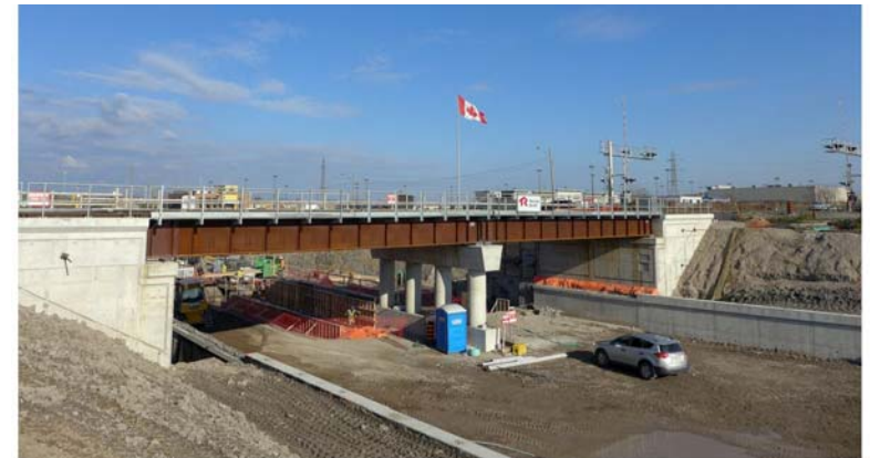
EXPANSION OF THE CENTENNIAL PARKWAY BRIDGE
