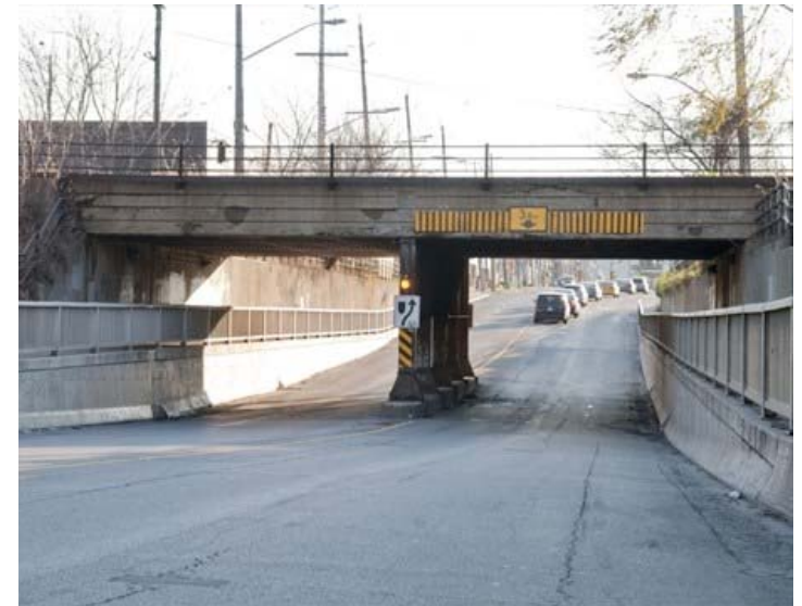
Kenilworth Ave. Bridge
